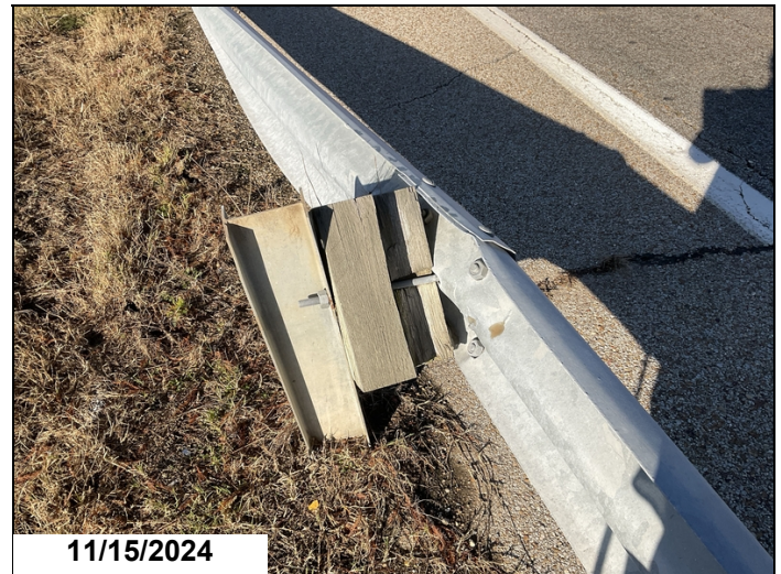
Bent 1 right approach rail wood spacer block damage 11-15-2024
