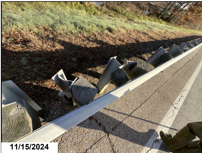
Bent 4 left approach rail wood spacer block damage 11-15-2024
